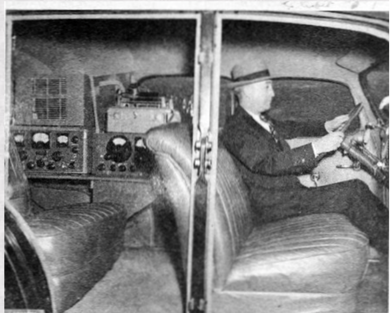
RID mobile intercept and direction finder unit used to home-in on clandestine radio activity.
